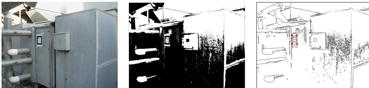
Fig. 3. (a) An input image of an exterior industrial setting, with a TriCode placed amongst other objects. The purpose here is to provide real-time data for AC ducts. (b) After conversion to bilevel. (c) Edges are marked as the boundaries of contiguous black areas. One chain of edges has its corners marked, indicating that it is the right shape and size to be passed to the identification process.
